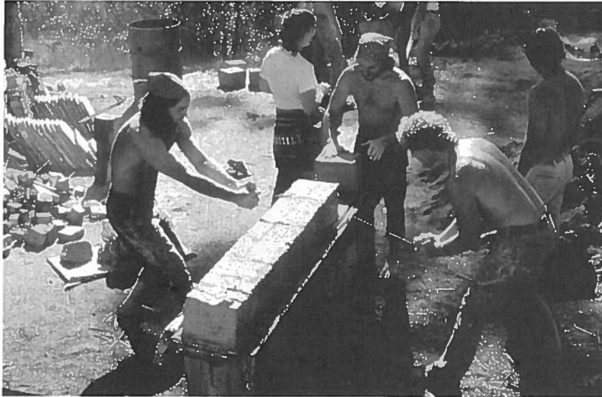
Fig 2—39: Brick making in trough mold, cut and sun dried.
