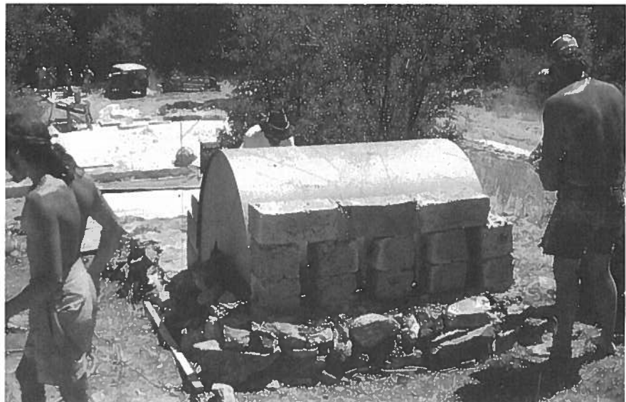
Fig 2—40: Start of straight wall with flue holes.
