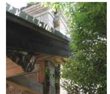
One of two large traditional massive stone buildings housing the Mashiko Sankokan (Hamada Shoji Reference Collection Museum) with severe damage from shifted walls caused by the earthquake. These historical buildings will have to be completely rebuilt, and likely will not be repaired for well over a year or more.
