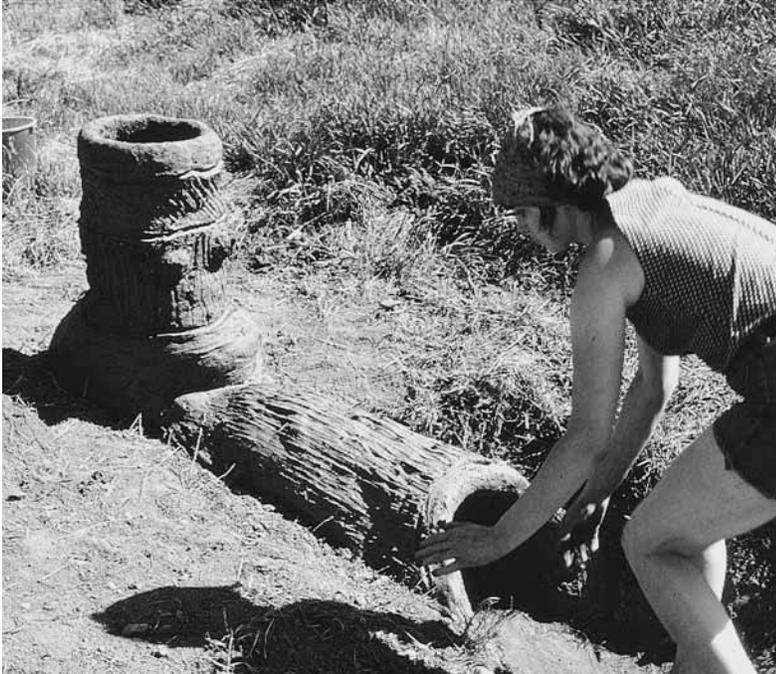
**A wood-fired raku kiln built from a mixture of fireclay, sandy gravel and sawdust.**
