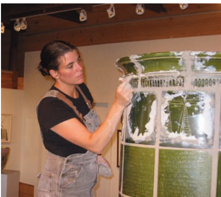
As the rows of kacheln are set, Steinhäuser removes wooden spacers and finishes the outside mortar joints. Excess mortar is removed with a sponge.
