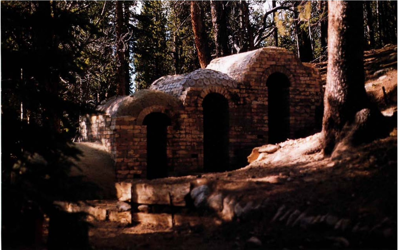
View of the newly built noborigama prior to adding stack and mudding the exterior.
