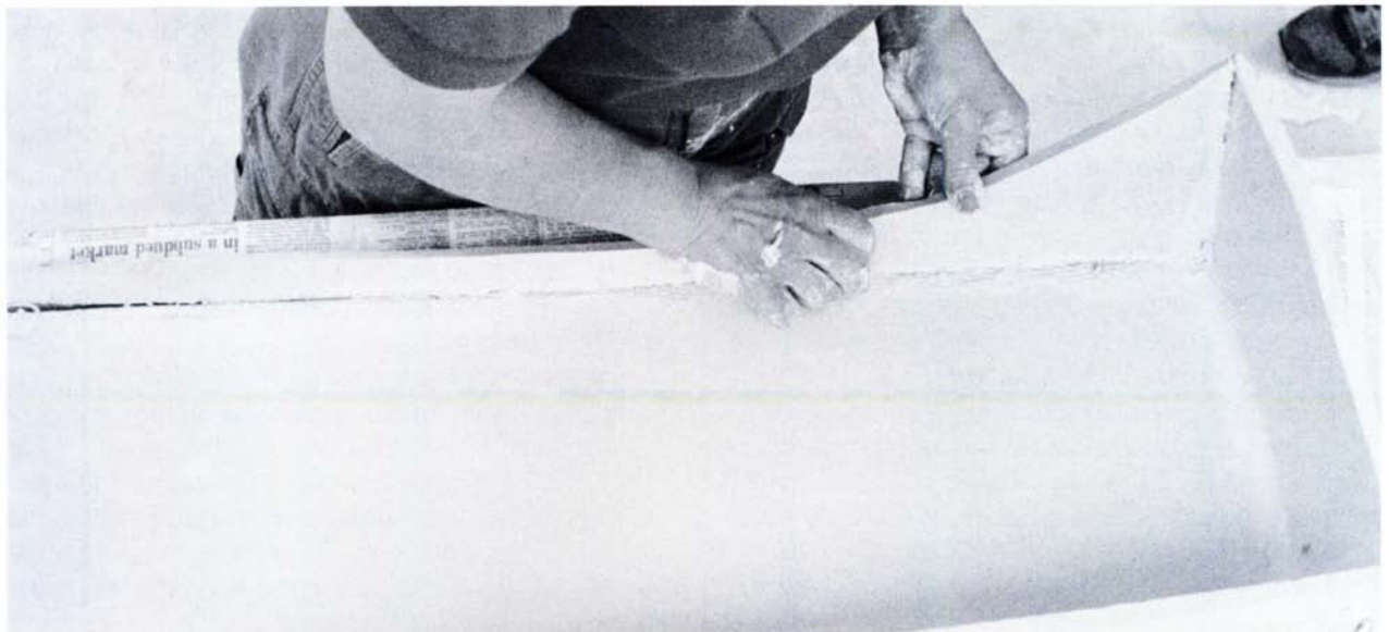
Construction of the lower left section of a fireplace commission. Slabs were carefully worked into place; they must be well attached to avoid cracking later.
