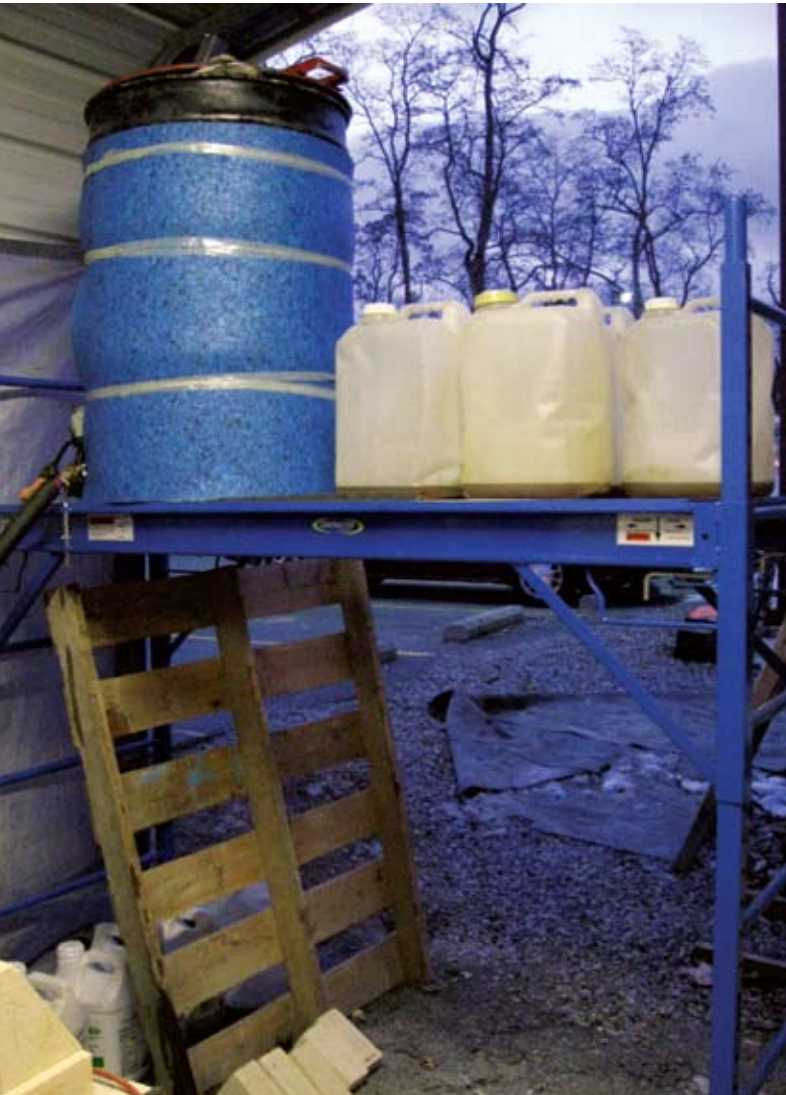
Shippensburg University's drip feed system for Waste Vegetable Oil (WVO) is fed by a barrel placed several feet above the burner height to allow for a gravity feed.
