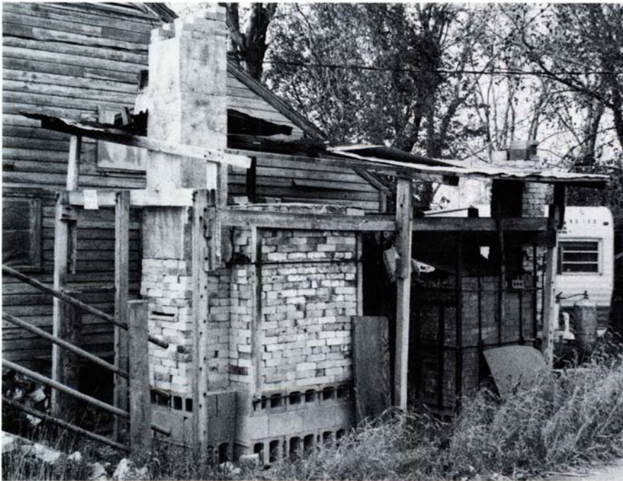
Alan Webster's salt kiln (foreground) with cast chimney
