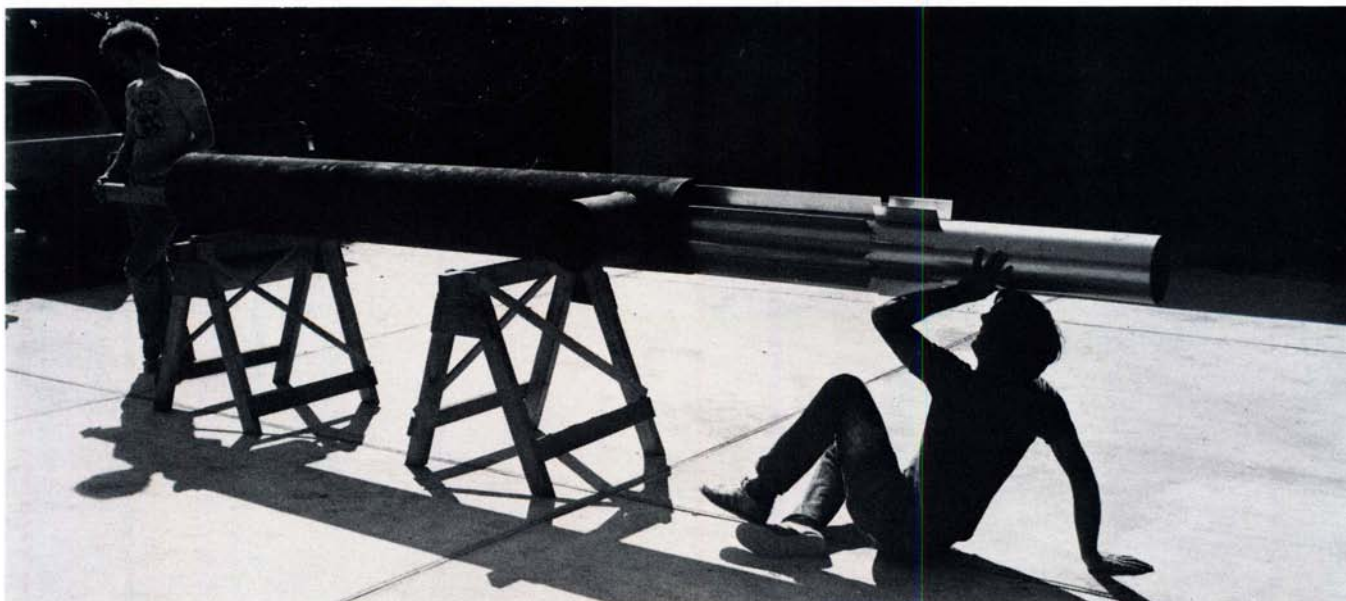
The stainless steel flue—four tightly fitted sections—is slid into its jacket.
