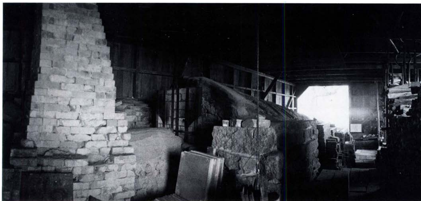
Top and above Richard Bresnahan's 40-foot naborigama (a chambered, climbing kiln) was constructed with salvaged granite from a school, firebrick from a brickworks and old incinerators.
