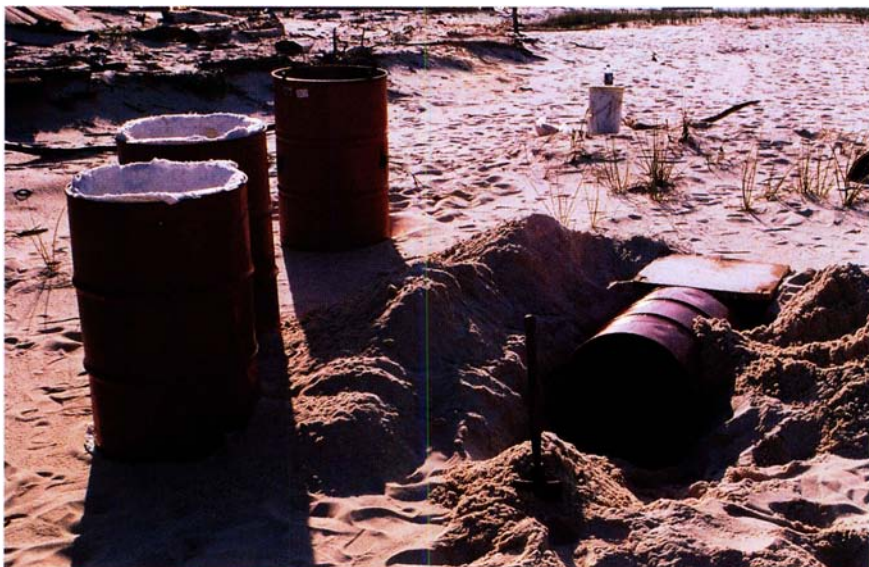
The Horn Island wood-burning kiln was constructed from three steel drum barrels. A trench was dug in the sand for the firebox barrel; the kiln shelf at the rear of the barrel will serve as the floor of the ware chamber barrel.
