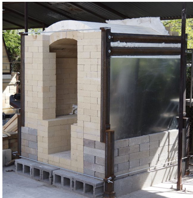
Opposite: Octagonal jar, 10¼ in. (26 cm) in height, iron-rich clay, wood and salt fired to cone 9–10, reduction cooled, 2018. Above: Reduction cooling gas kiln building in progress at Ohio University in Athens, Ohio, 2021. Below: Hayun Surl with Monument , 5 ft. 6 in. (1.7 m) in height, iron-rich clay, salt fired to cone 7, 2020.
