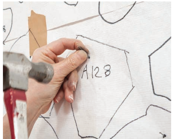
6. Nailing right through the tough Tyvek template.
