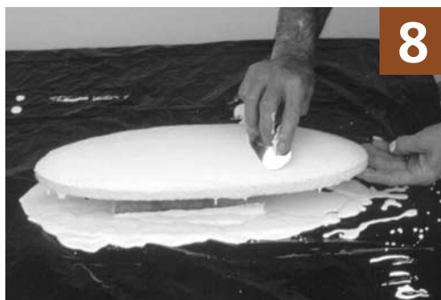
Smooth plaster with metal rib.
