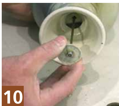
10 Slide the other end of the rod into the bottom opening, through the bottom guide and into the handle.
